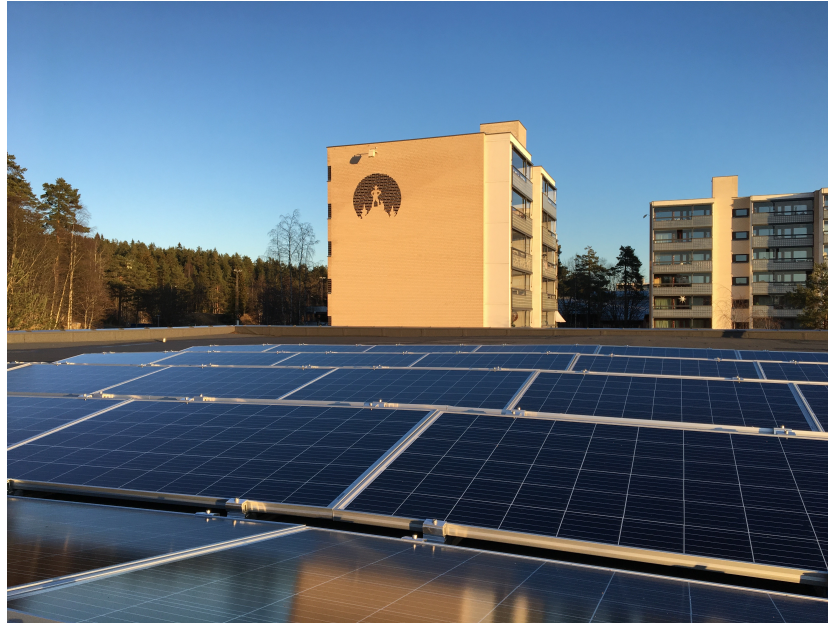
Figure 11: Photovoltaic panels on the garage roof at Røverkollen
