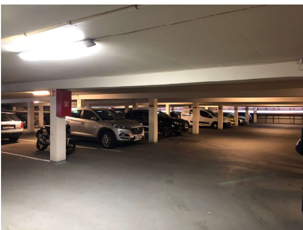
Figure 6 The four-storey parking garage at Røverkollen
