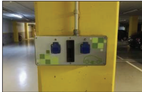
Figure 2: Charging point in Eurecat premises
