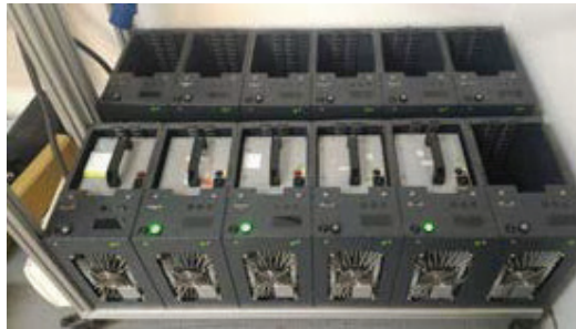
Figure 3-11: Battery hub in MOTIT premises
