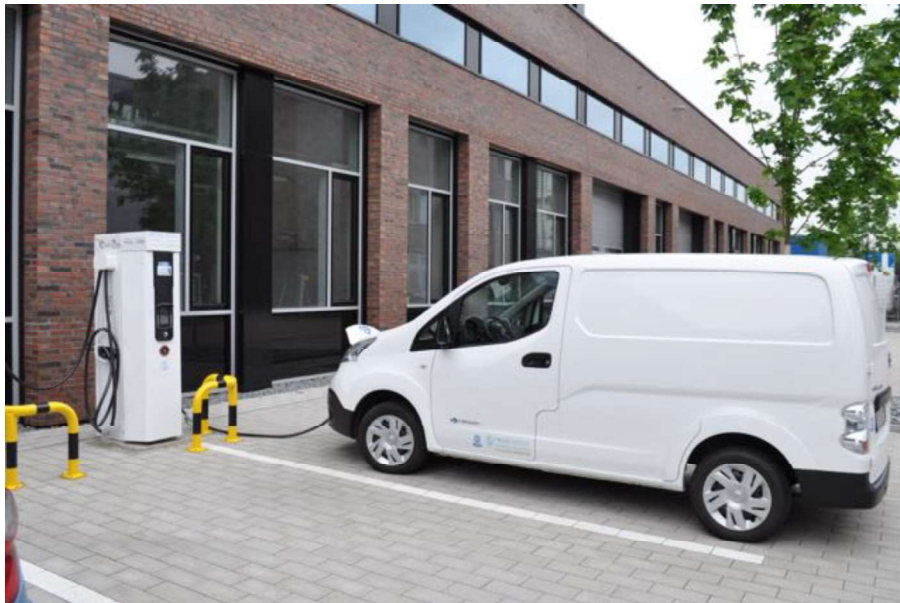
Figure 19: Electric car recharging on CS#4
